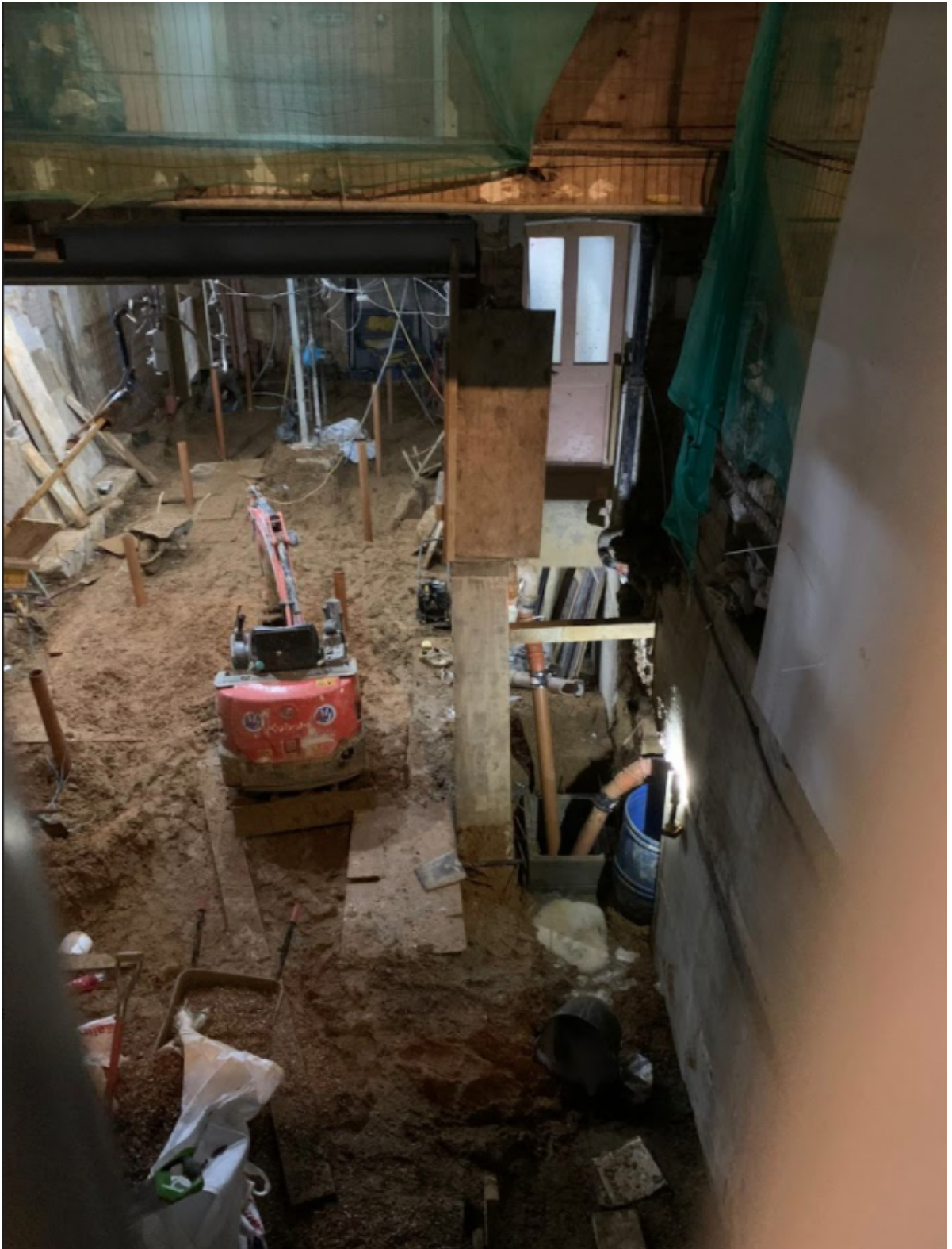
Recent photo of basement works:
